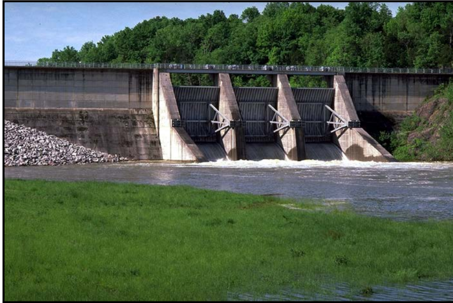
Figure 3: Tellico Dam (Photo by TVA)
