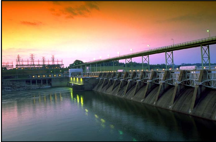
Figure 1: Fort Loudoun Dam (Photo by TVA)
