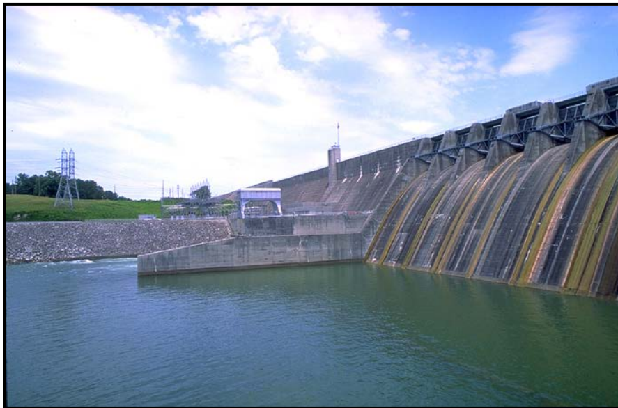
Figure 2: Cherokee Dam (Photo by TVA)
